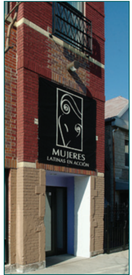
THE MUJERES BUILDING'S ENTRANCE FACES A BUSTLING RESIDENTIAL AND COMMERCIAL STREET.
