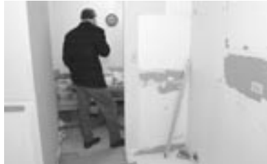
SERAFIMA'S "RIPPED OUT" KITCHEN
